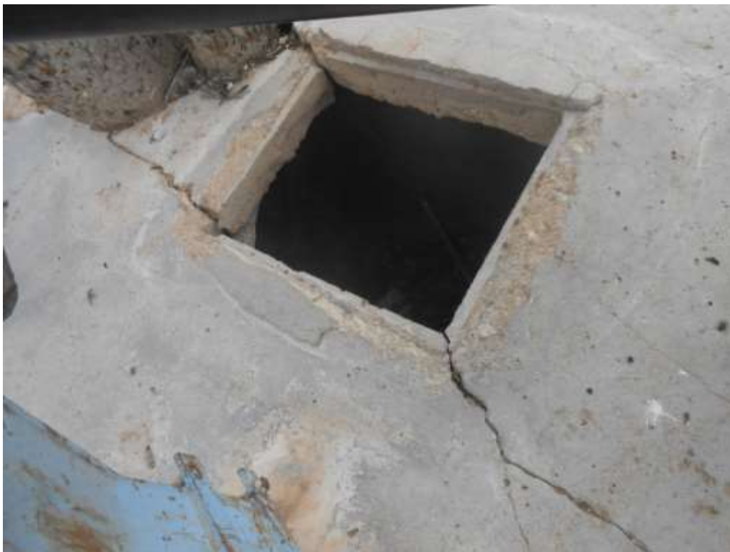
The dry well in February this year (2025)
